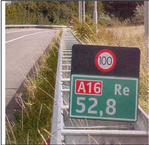
A hectometre post with speed limit reminder at motorways in the Netherlands
