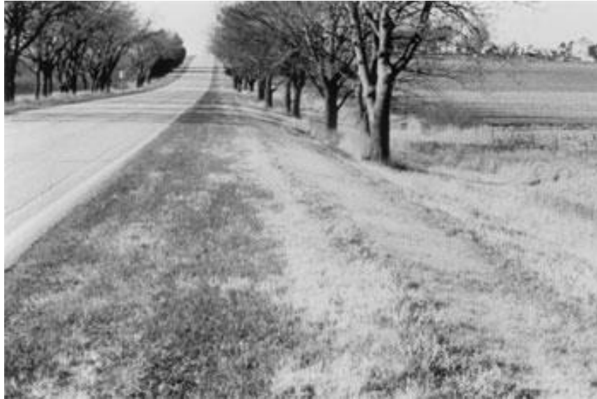
Figure 3.14: Typical Roadway with Roadside Hazard Rating of 5: Clear zone between 5 and 10 ft; side slope about 1V:3H, virtually non-recoverable (Source: AASHTO, 2010)
