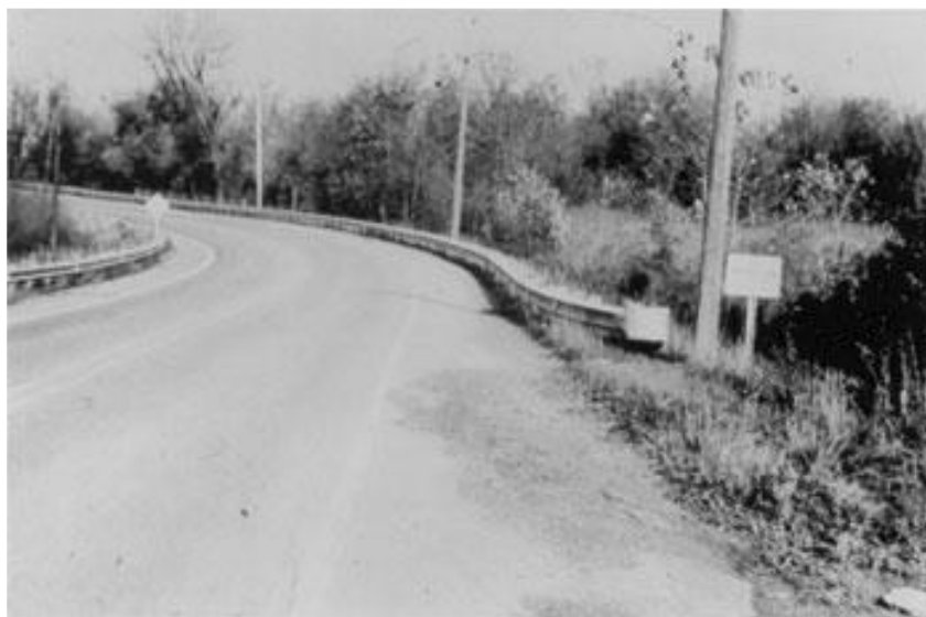
Figure 3.13: Typical Roadway with Roadside Hazard Rating of 4: Clear zone between 5 and 10 ft; side slope about 1V:3H or 1V:4H, marginally forgiving, increased chance of reportable roadside crash (Source: AASHTO, 2010)
