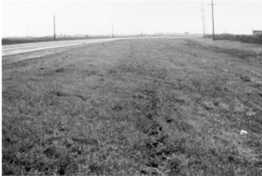
Figure 3.10: Typical Roadway with Roadside Hazard Rating of 1: Clear zone greater than or equal to 30 ft side slope flatter than 1V:4H, recoverable (Source: AASHTO, 2010)
