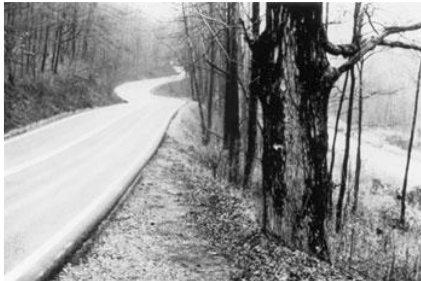
Figure 3.15: Typical Roadway with Roadside Hazard Rating of 6: Clear zone less than or equal to 5 ft; side slope about 1V:2H, non-recoverable (Source: AASHTO, 2010)
