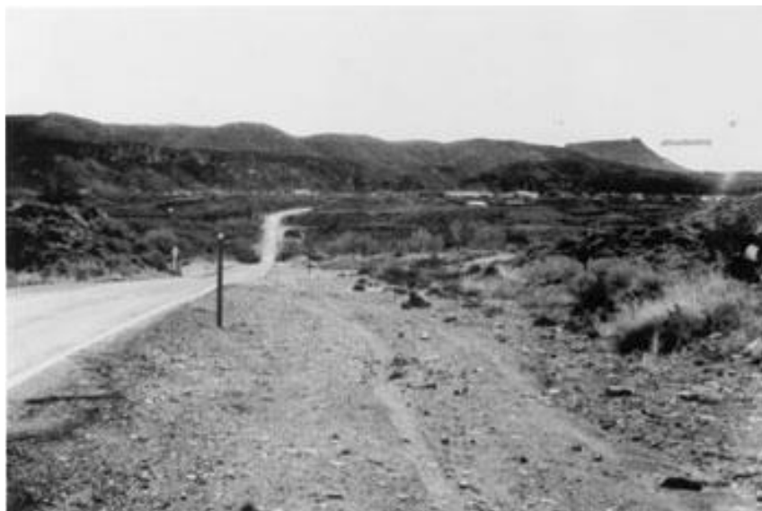
Figure 3.11: Typical Roadway with Roadside Hazard Rating of 2: Clear zone between 20 and 25 ft; side slope about 1V:4H, recoverable (Source: AASHTO, 2010)
