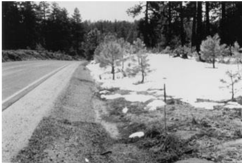
Figure 3.12: Typical Roadway with Roadside Hazard Rating of 3: Clear zone about 10 ft; side slope about 1V:3H, marginally recoverable (Source: AASHTO, 2010)
