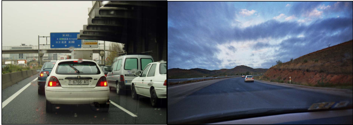
Figure 2. Examples of serious road infrastructure deficiencies. To the left: a concrete cornice obscuring the view of an informative traffic sign in one of the most travelled motorways in Spain. To the right: total absence of road markings after repaving the motorway connecting Madrid and Barcelona in Spain.
